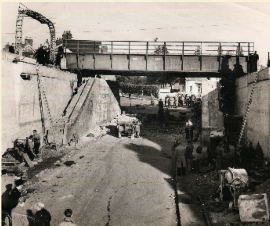
View looking up Station Road, January 1960. The bridge was being widened to accommodate additional track.
