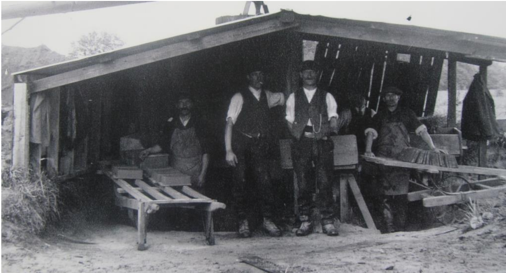
This is where the bricks were moulded. They would then be dried before going to a kiln to be fired.
