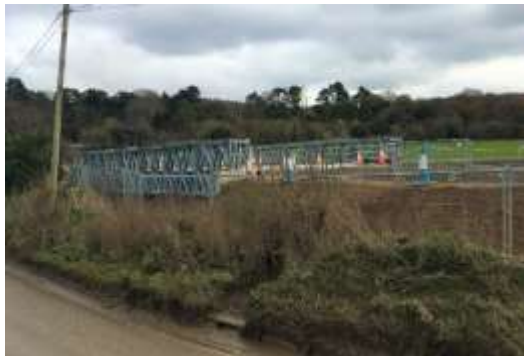
HS2 are constructing a ventilation vent in this valley. This bridge takes construction vehicles over the river.
