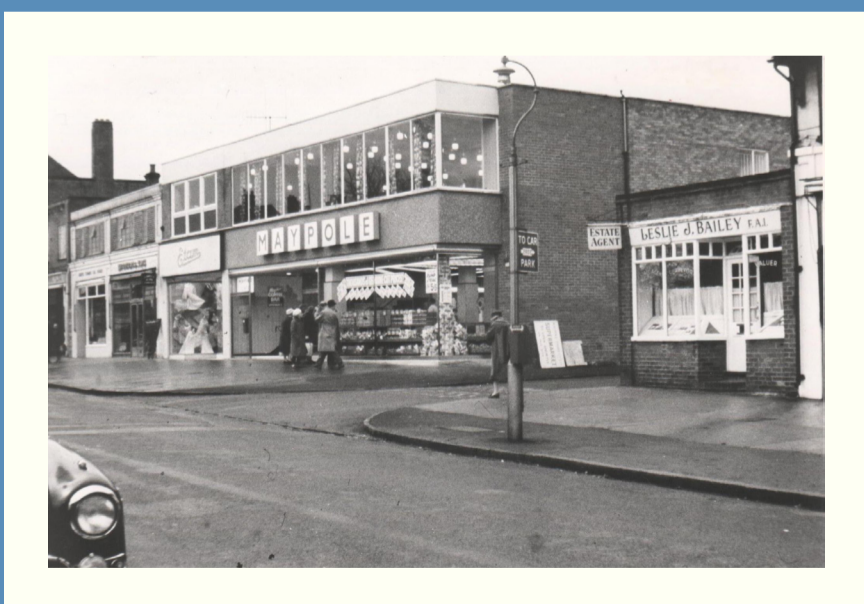
Maypole, Amersham's first self-service supermarket, which opened in 1962
